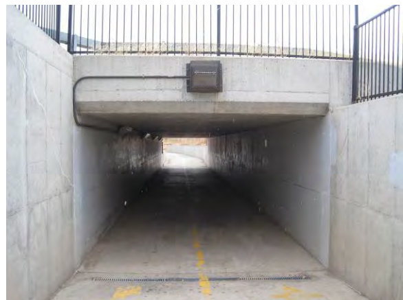
Figure 14. Undercrossings, such as this one located at College Drive on the Dry Creek Greenway, provide a comfortable crossing by separating bicyclists from motorists.
