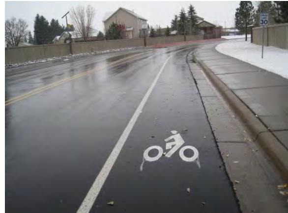
Figure 6. Bicycle lanes, such as these facilities on Vandehei Avenue, provide a measure of separation between cyclists and motor vehicles.
